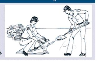
Fold over the open end of the bag in a triangle to prevent sand from leaking out. Close-knit burlap bags are recommended.
